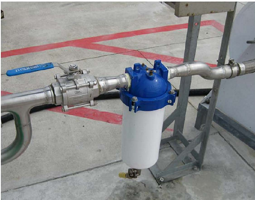
Figure 2 - Variant 7 - Typical External Filter Installation
